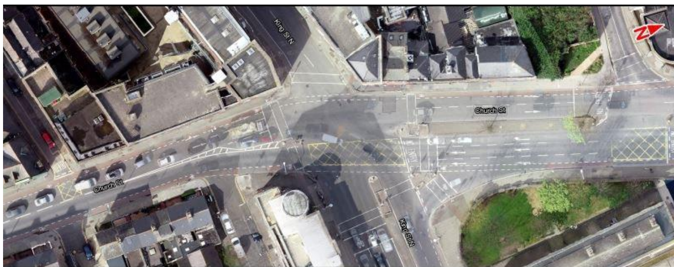
Image 6.20: R108 Church Street Upper / R804 King Street North / R108 Church Street Four-Arm Signalised Junction
