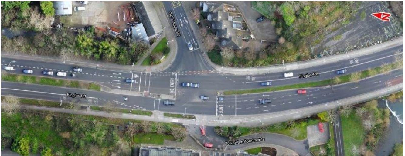
Image 6.28: R135 Finglas Road / Access to Tolka Vale Apartments / R102 Old Finglas Road Four-Arm Signalised Junction
