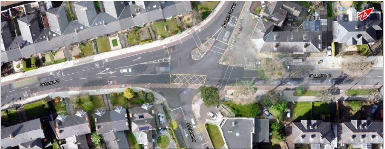
Image 6.10: R108 St. Mobhi Road / Botanic Road / Fairfield Road / R108 Botanic Road Four-Arm Signalised Junction
