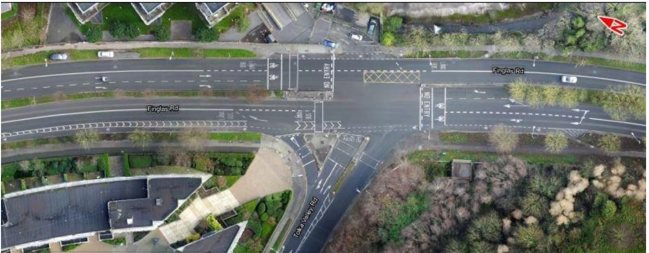
Image 6.27: R135 Finglas Road / R102 Tolka Valley Road / Four-Arm Signalised Junction
