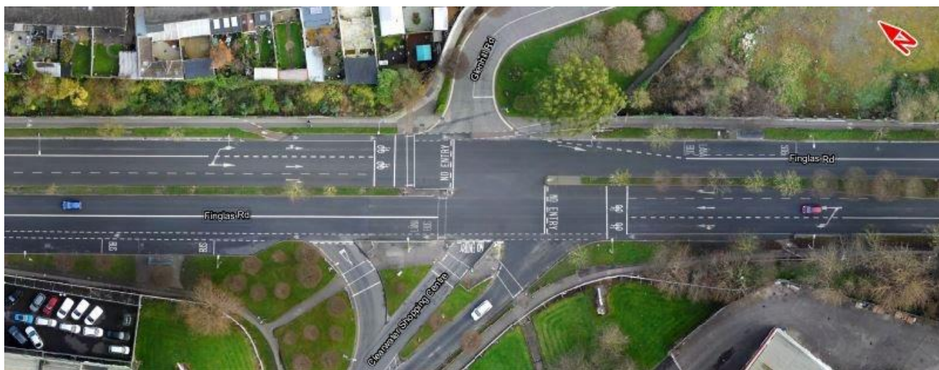
Image 6.25: R135 Finglas Road / Clearwater Shopping Centre / Glenhill Road Four-Arm Signalised Junction
